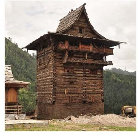
132(a-c). Tower temples. Tower with a square base and cantilevered upper storey built in kath-khuni fashion are typical to western Himalayas. The deity is placed at the highest level at the top, the other floors are used to store grain for the pujari and for the villagers. a. Temple at Balag; b. Temple at Chopal; c. Temple at Pujarli 7.
