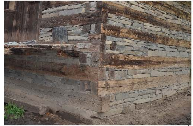
88(a-b). Examples of kath-khuni corner junctions. a. Wall corner of Bara-kila tower temple at Chitkul; b. Corner junction of a house in Gavas.
