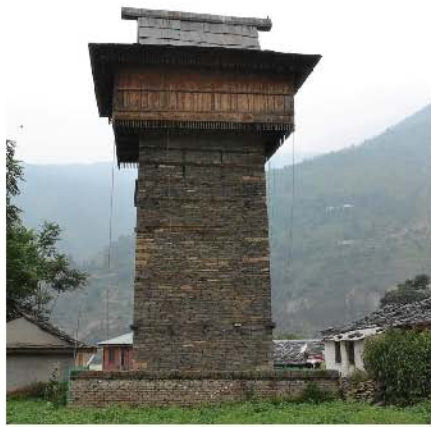
132(a-c). Tower temples. Tower with a square base and cantilevered upper storey built in kath-khuni fashion are typical to western Himalayas. The deity is placed at the highest level at the top, the other floors are used to store grain for the pujari and for the villagers. a. Temple at Balag; b. Temple at Chopal; c. Temple at Pujarli 7.
