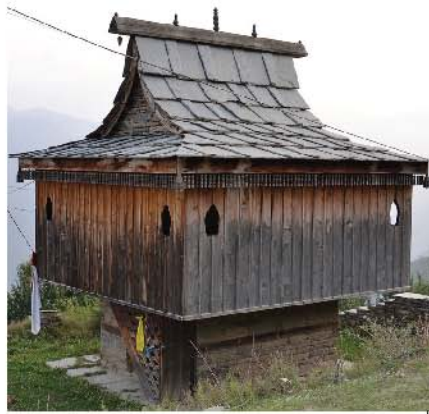
132(a-c). Tower temples. Tower with a square base and cantilevered upper storey built in kath-khuni fashion are typical to western Himalayas. The deity is placed at the highest level at the top, the other floors are used to store grain for the pujari and for the villagers. a. Temple at Balag; b. Temple at Chopal; c. Temple at Pujarli 7.
