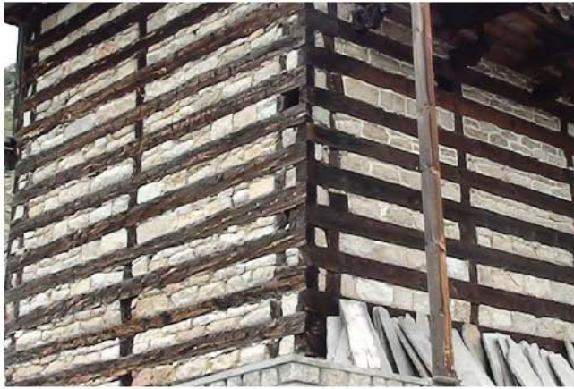
88(a-b). Examples of kath-khuni corner junctions. a. Wall corner of Bara-kila tower temple at Chitkul; b. Corner junction of a house in Gavas.
